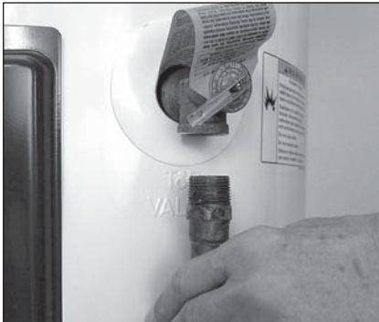
Figure 11 - Removing the T&P Relief Valve discharge pipe.
