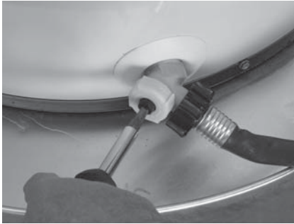
Figure 10 - Draining the old water heater.
