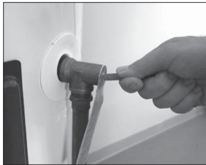
Figure 38 - T&P Relief Valve
