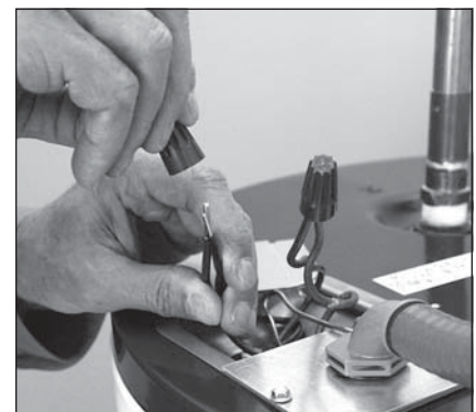
Figure 19 - Connecting the electrical wires.
